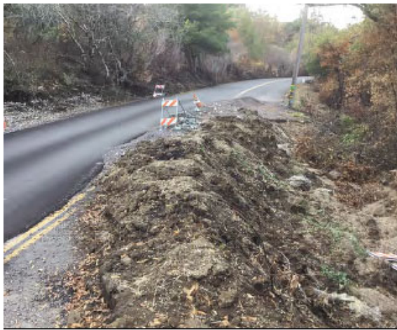
Photo 29: Evidence of road washout; fill material and straw placed on the hillside to prevent further material loss.
